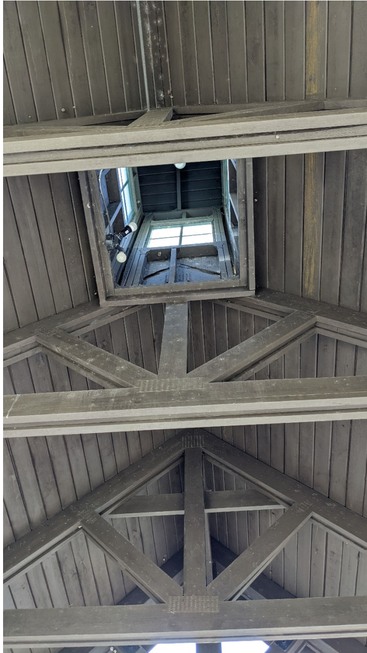
Photograph No.9 – View of wood trusses
