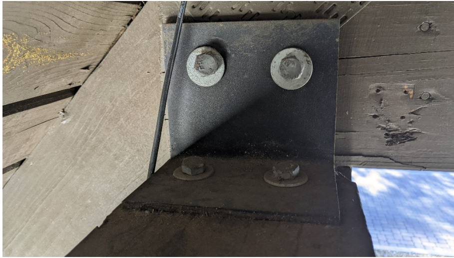
Photograph No.7 – Typical truss tie-down
