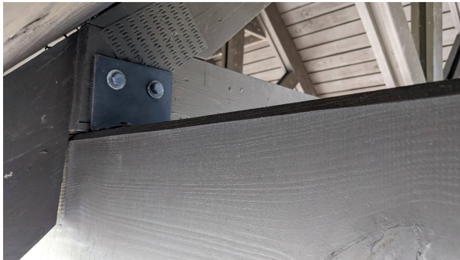
Photograph No.8 – Typical truss tie-down
