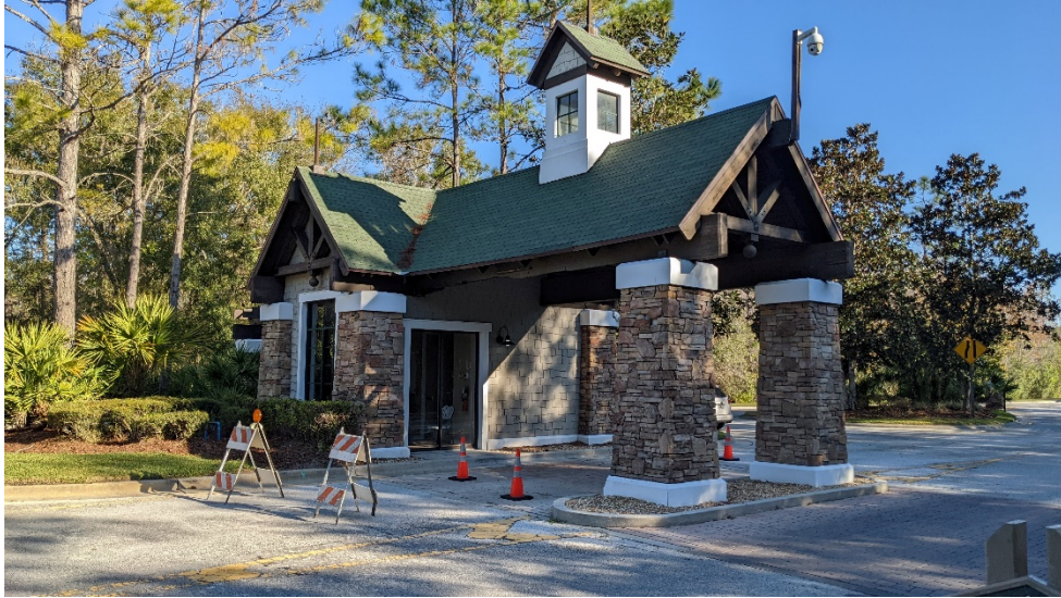
Photograph No.1 –View of Ranger Station
